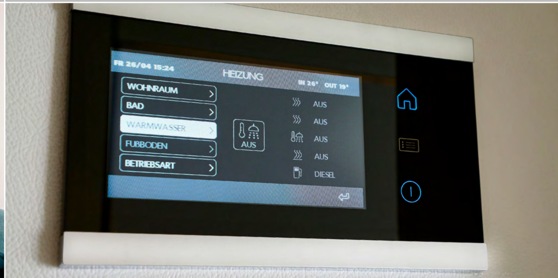
Hot water heating on diesel (Eberspächer 5 kW) dual zone Control unit with touch-display for controlling and monitoring of all components
